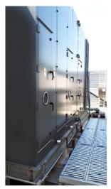
Thermo-Composites units including high efficiency Sensible Wheel Exchanger, Evaporative Cooler and Indirect Gas Burner
